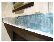
REMOVE ALUMINUM, CALK, PEEL AND STICK MEMBRANE TAPE, ALUMINUM CLEAT AND FASTENERS, ALL ADHESIVE / ADHESIVE RESIDUE AND COATINGS DOWN TO CONCRETE ON ALL LEDGES.
